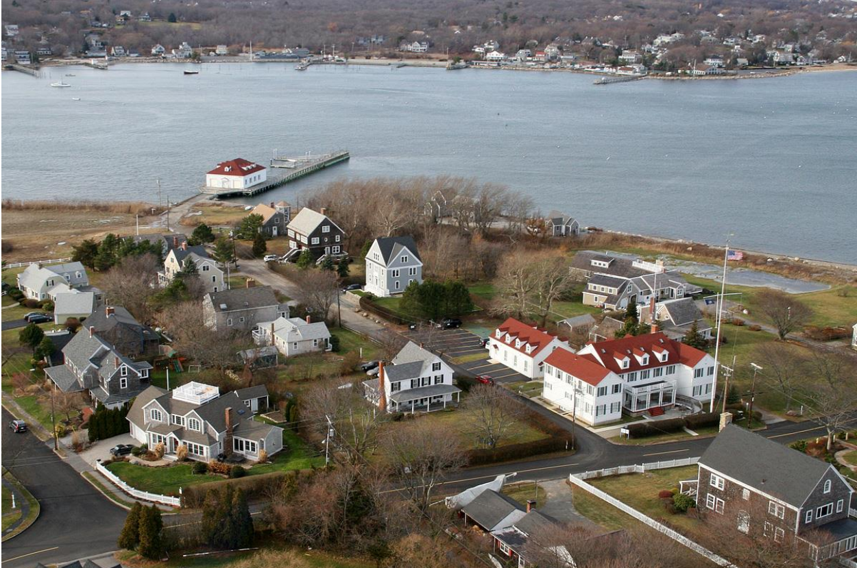
Figure 3.18. The headquarters office for SBNMS is located in Scituate, Massachusetts. The campus is composed of an administrative building, meeting annex, and a marine operations center on the waterfront where the R/V Auk is berthed (buildings with red roofs). Sanctuary staff along with other local, state, and federal partners are housed in the administrative building. Source: Microsoft Corporation/Pictometry International Corp., 2006
