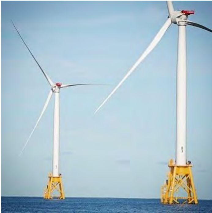
Figure 3.8. SBNMS will identify, evaluate, and track potential compatible uses, such as offshore wind projects. This photo is of Block Island Wind Farm off Rhode Island. Photo: Rhode Island Sea Grant
